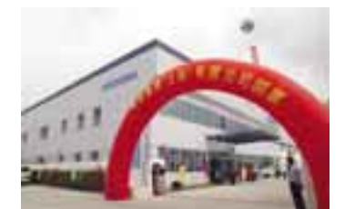
Second Production Plant in Shanghai, China
