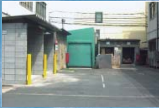
Recycling platform (temporary separation)
